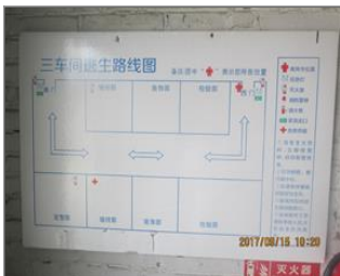
Photo of fire safety equipment Evacuation map.JPG
