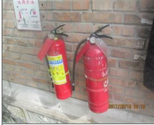
Photo of fire safety equipment Fire extinguishers.JPG
